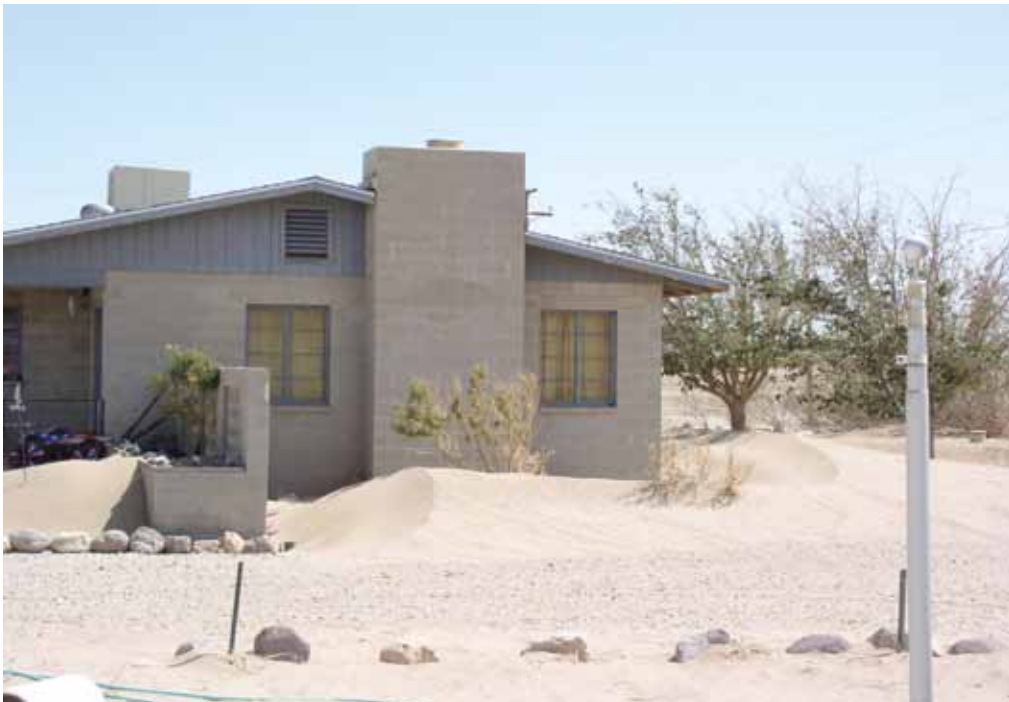
Figure 4: This residence experienced blown sand deposits in an unstable landscape.
